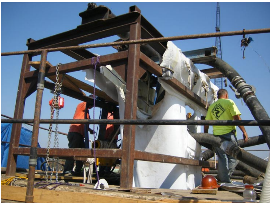
Water is being filled in the inverted liner.
